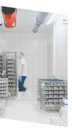
Optimizing cold room cleaning procedures can significantly improve efficiency and reduce energy consumption. Heating cold rooms prior to washdown minimizes the formation of fog and condensation, streamlining the cleaning process and reducing the risk of water damage. Following cleaning, promptly exhausting the moist, warm air before initiating the cool-down phase reduces the energy required for refrigeration.
