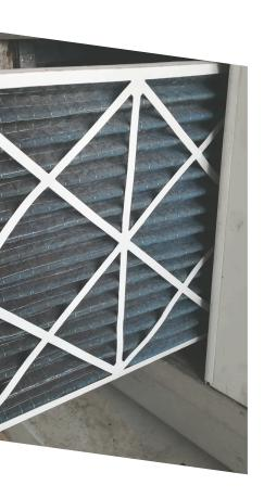
Maintaining sufficient air turnover within a bakery is critical for removing airborne contaminants that can compromise product quality and safety. This is achieved through adequate air exchange rates, measured in air turns per hour, which effectively dilute and remove particles and microorganisms. Complementing air turnover, and appropriate filtration levels, quantified by Minimum Efficiency Reporting Value (MERV) ratings, are essential.
